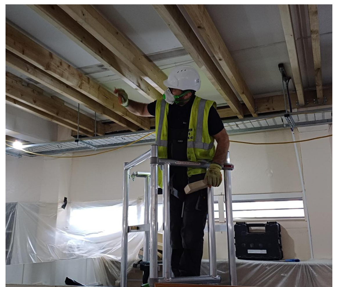
Joists being installed to support RAAC
